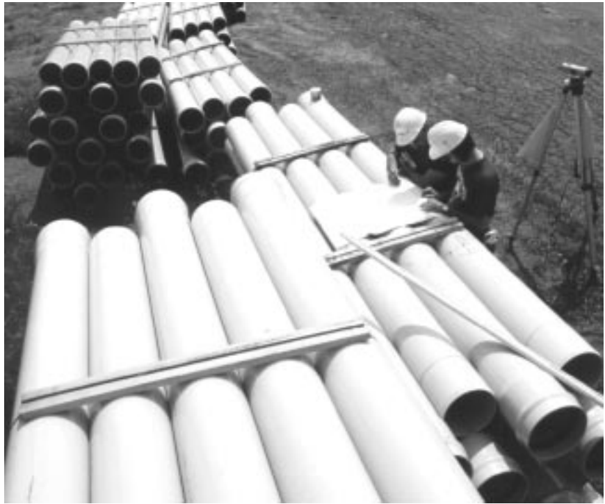
Fig. 2.1: AQUALOC pressure pipe on the job site
