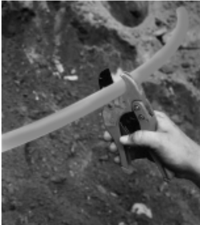
Fig. 4.1: Cut MUNICIPEX with approved tool
