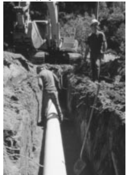
Fig. 2.8: Installation of AQUALOC pressure pipe
