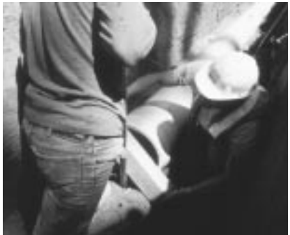
Fig. 1.1: Installing AQUALOC pressure pipe
