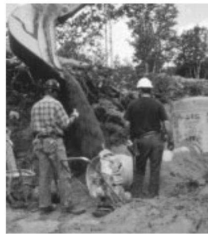
Fig. 3.2: RAURIB being installed in a sanitary sewermain
