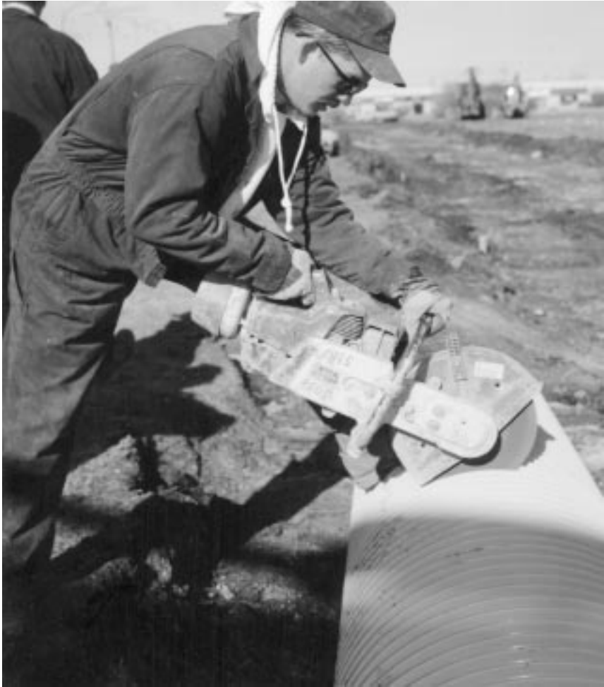
Fig. 1.5: Installation is made even easier by the ability to cut RAURIB in the field.
