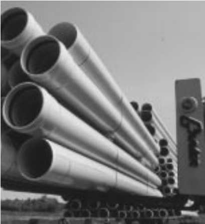
Fig. 3.7: Unloading DURALOC sewer pipe on a jobsite
