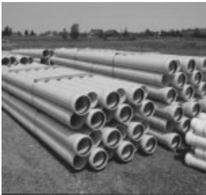
Fig. 2.6: Storage of PVC pipe
