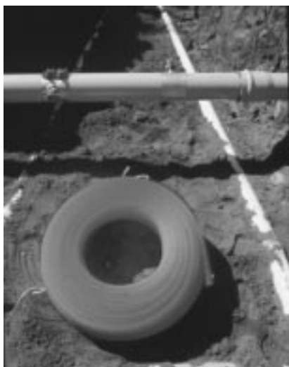
Fig. 4.1: MUNICIPEX on job site ready for installation
