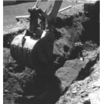
Fig. 3.9: Backfilling DURALOC sewer pipe
