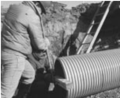
Fig. 1.3: Installing RAURIB sewer pipe
