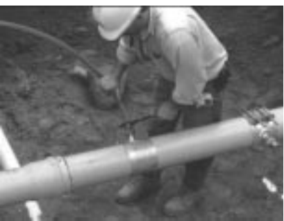
Fig. 1.4: MUNICIPEX service installation
