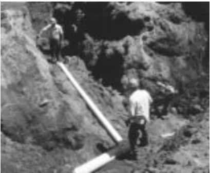
Fig. 1.2: DURALOC sewer pipe lateral installation
