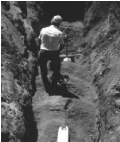
Fig. 3.1: Tamping of backfill during installation of DURALOC sewer pipe
